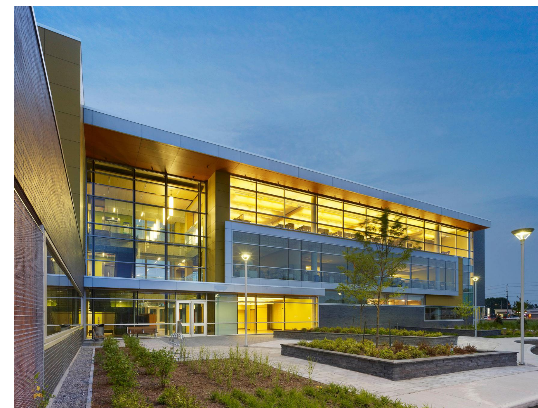
The James Bartleman Archives & Library in Ottawa, designed with both passive and mechanical systems: http://www.sabmagazine.com/blog/2014/03/24/james-bartleman-archives-library-materials-centre/
